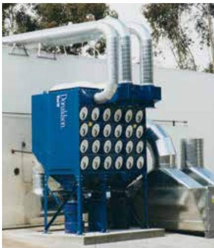
DFO on Metal Grinding 31,000 cfm (52,658 m 3 /h)
