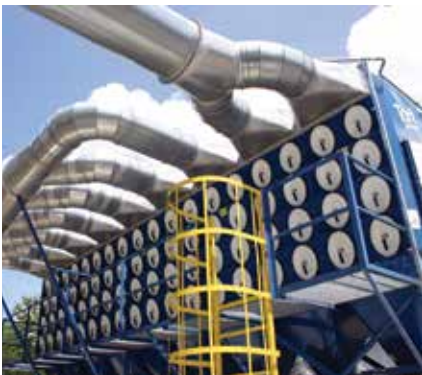
DFO on Sawdust 57,500 cfm (97,692 m 3 /h)
