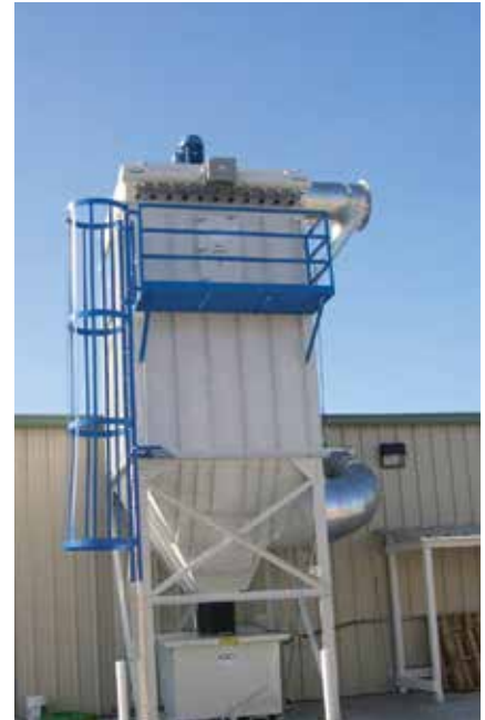
FS on Woodworking 20,000 cfm (33,973 m 3 /h)
