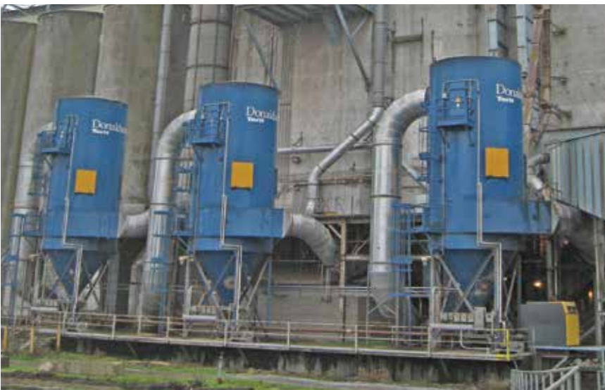
RF - Grain Terminal 61,000 cfm (103,618 m 3 /h)
