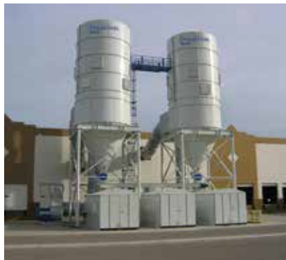
LP on Wood Dust 160,000 cfm (271,784 m 3 /h)
