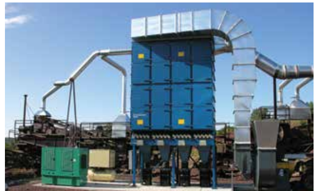
DLMC on Rock Crushing 41,000 cfm (69,645 m 3 /h)
