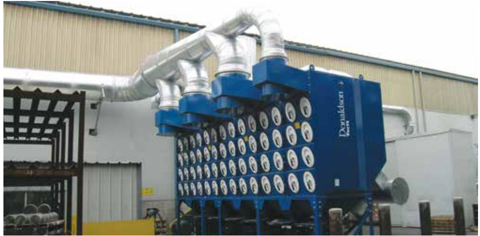
DFO on Grinding 74,000 cfm (125,700 m 3 /h)
