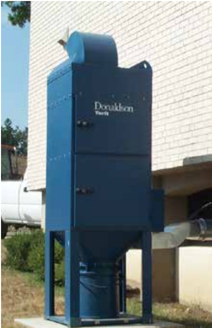
UMA - School Wood Shop 2,000 cfm (3,397 m 3 /h)
