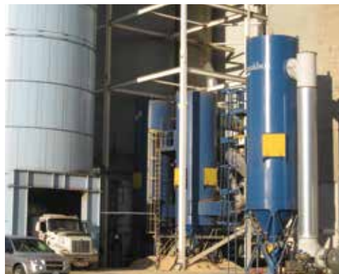
RF - Grain Terminal 34,000 cfm (57,754 m 3 /h)
