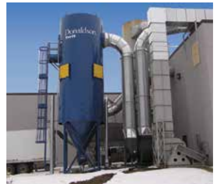
RF - Cabinet Shop 48,500 cfm (82,385 m 3 /h)
