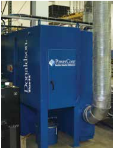
TG on Plasma Cutting 2,300 cfm (3,90 m 3 /h)
