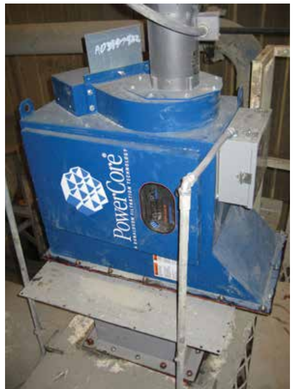
CPV - Feed Hopper 350 cfm (595 m 3 /h)
