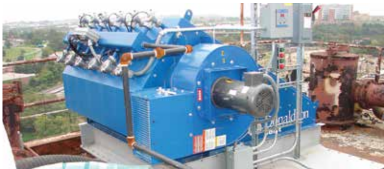
CPV - Multiple Cement Silos 4,800 cfm (8,154 m 3 /h)
