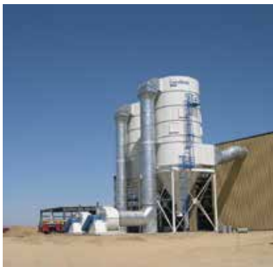
LP on Nut Dust 280,000 cfm (475,622 m 3 /h)
