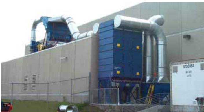
DLMC on Paper Dust 27,000 cfm (45,864 m 3 /h)
