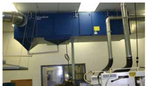
MODULAR MEDIAFILTER™ on Grinding 2,000 cfm (3,397 m 3 /h)
