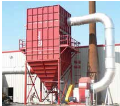
MB on Glass Processing 25,000 cfm (42,466 m 3 /h)
