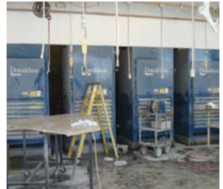
DWS on Granite Finishing 22,000 cfm (37,370 m 3 /h)
